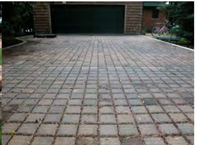
Dickinson Soil and Water Conservation District, Pervious Pavers
