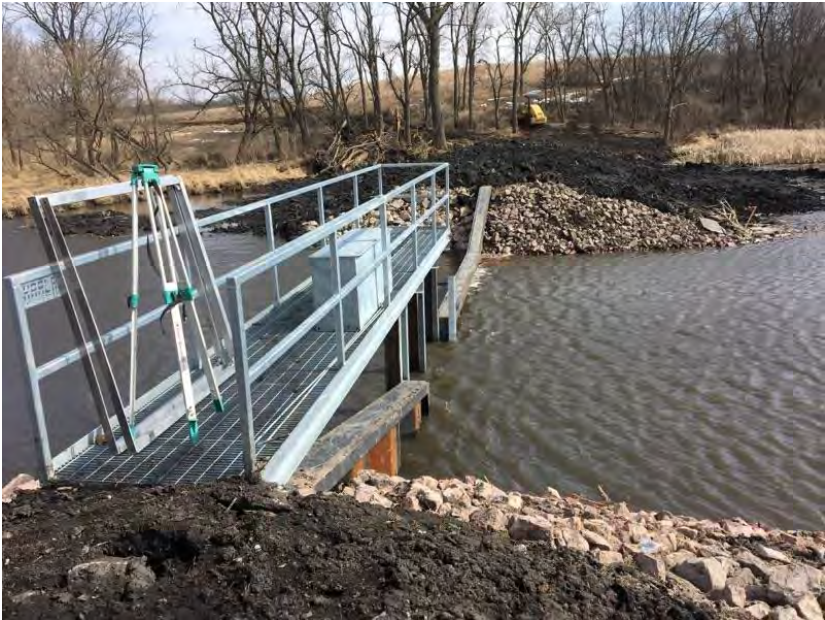
Little Swan Lake Restoration
