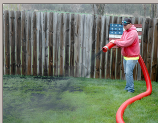
Pneumatic blower truck
